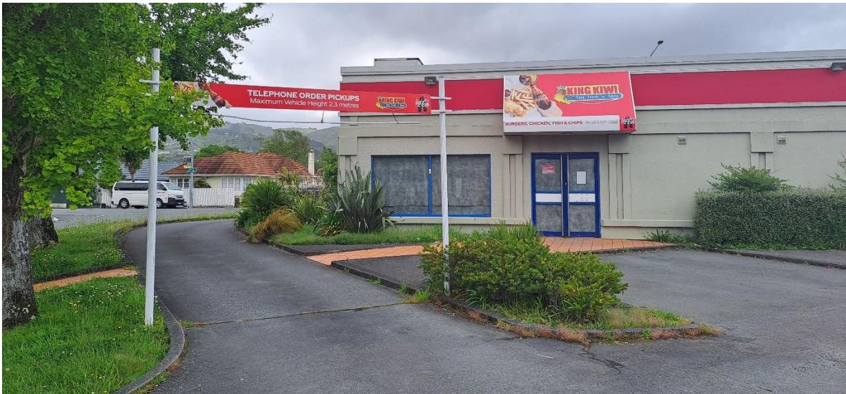
Figure 8 Entrance to the existing drive through and the existing façade.
