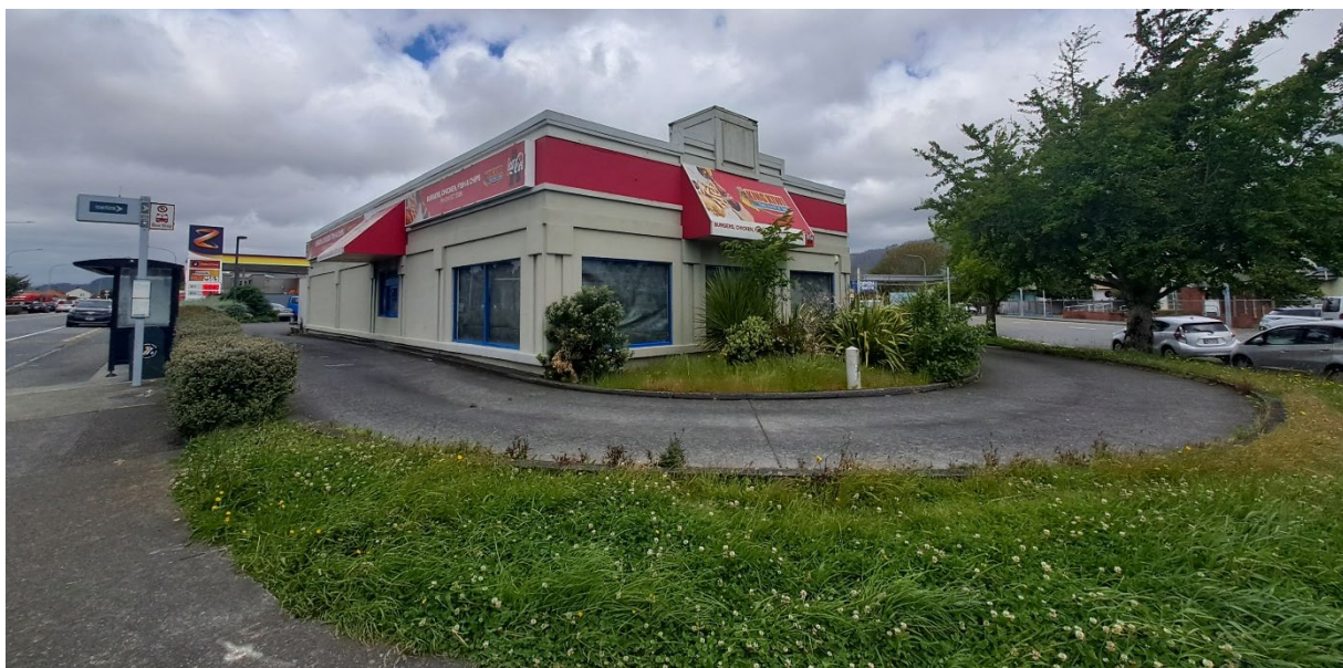
Figure 14 The existing drive through which is proposed to be widened to allow for better manoeuvring.
